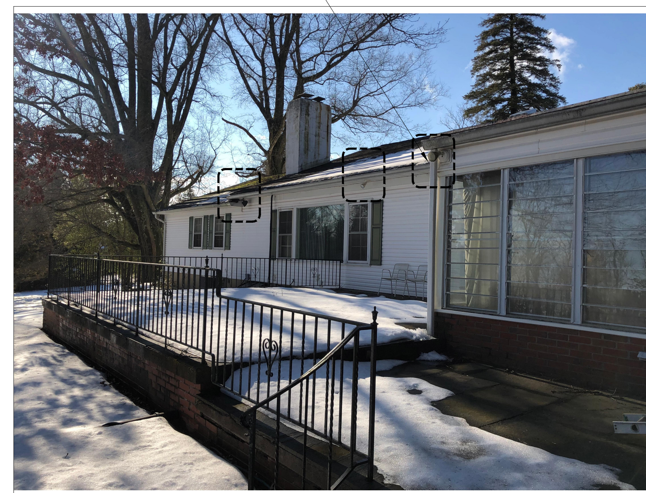
3 EXISTING REAR OF BUILDING N.T.S.
